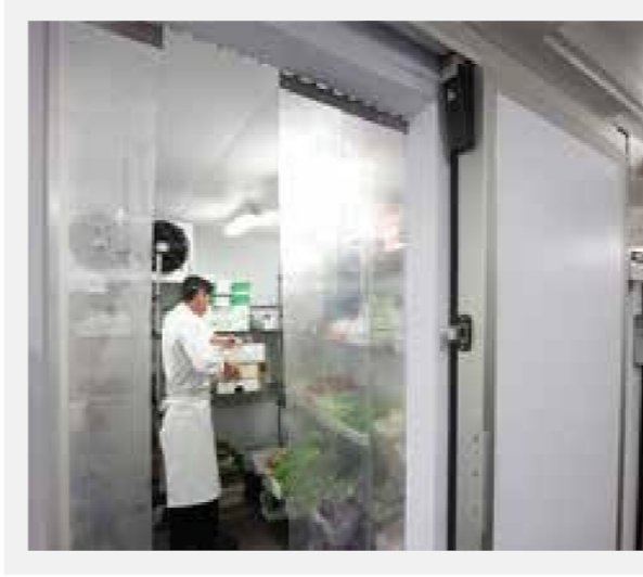
Cold Storage Freezer Rooms
